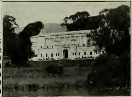
VIEW OF NEW MEMORIAL COLUMBARIUM (Largest and most beautiful Columbarium ever erected)
